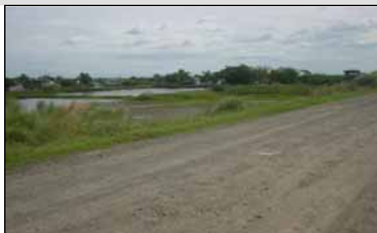
A newly-developed dike road
